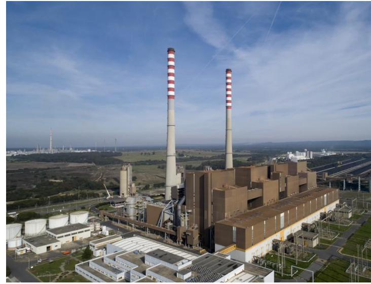
Sines Coal-Fired Thermoelectric Power Plant
